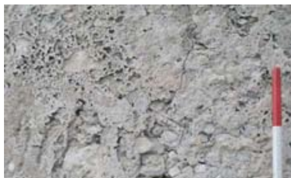
FIGURE 12. Cagliari, Su Perdusemi tower. Deterioration of the external plaster.
