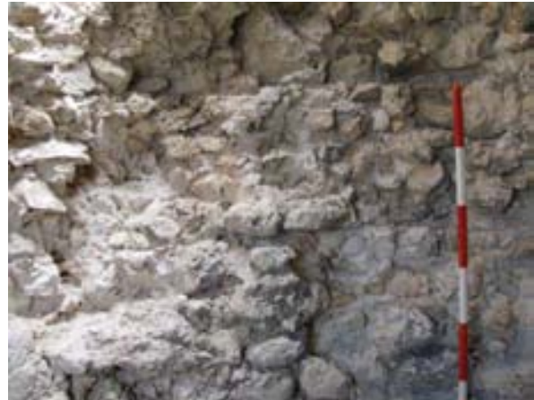
FIGURE 4. Cagliari, Su Perdusemmini tower. The picture shows the ‘cantieri’ masonry technique used.
