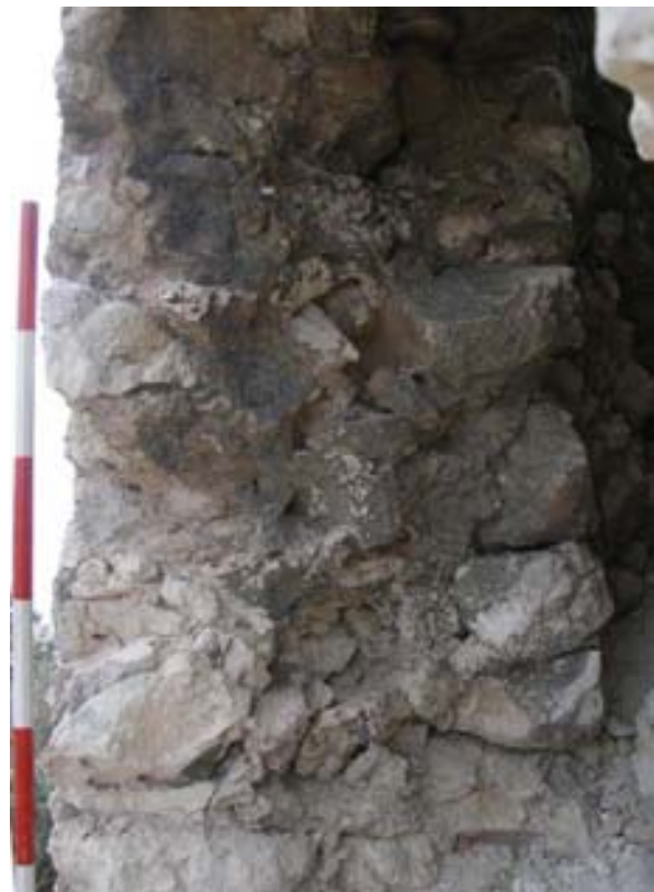
FIGURE 5. Cagliari, Su Perdusemmini tower. Vertical section of the masonry.
