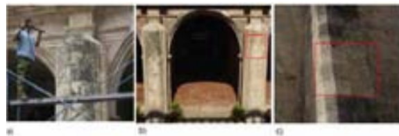
FIGURE 2. Hydrofuge products application. a) surfaces cleaning; b) column of courtyard north; c) column of northern facade.
