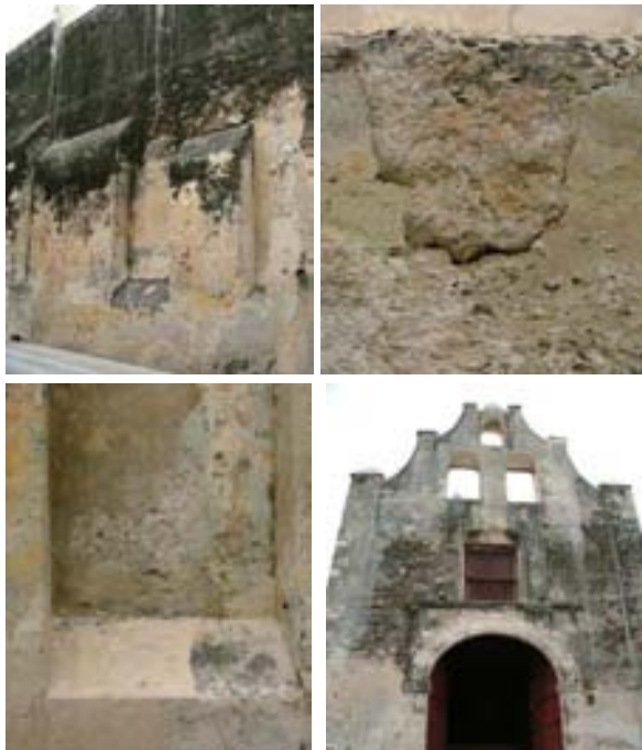
FIGURE 3. Several aspects of degradation phenomena in San Roque Church.
