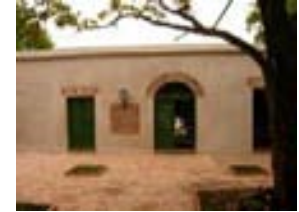
FIGURE 4. 1 st courtyard restored.
